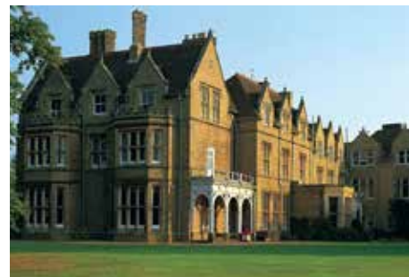
D South Building
